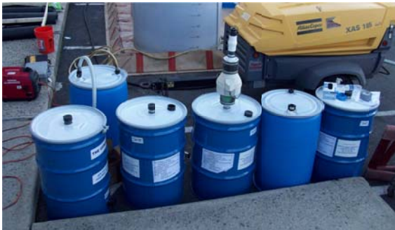
Photograph 3 - Odor Control System
