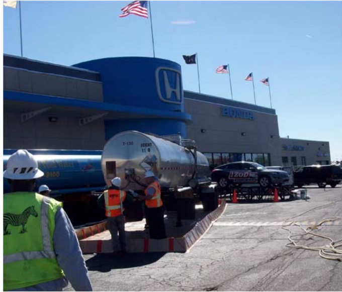
Photograph 2 - Portable Containment
