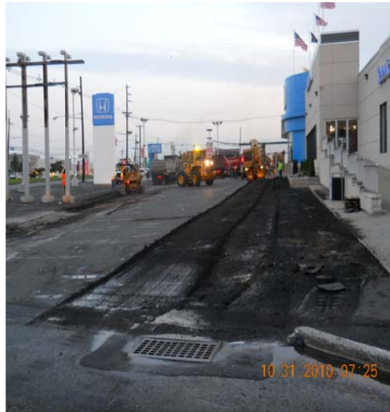
Photograph 7 - Pavement Milling
