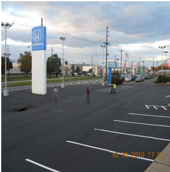
Photograph 8 - Pavement Striping
